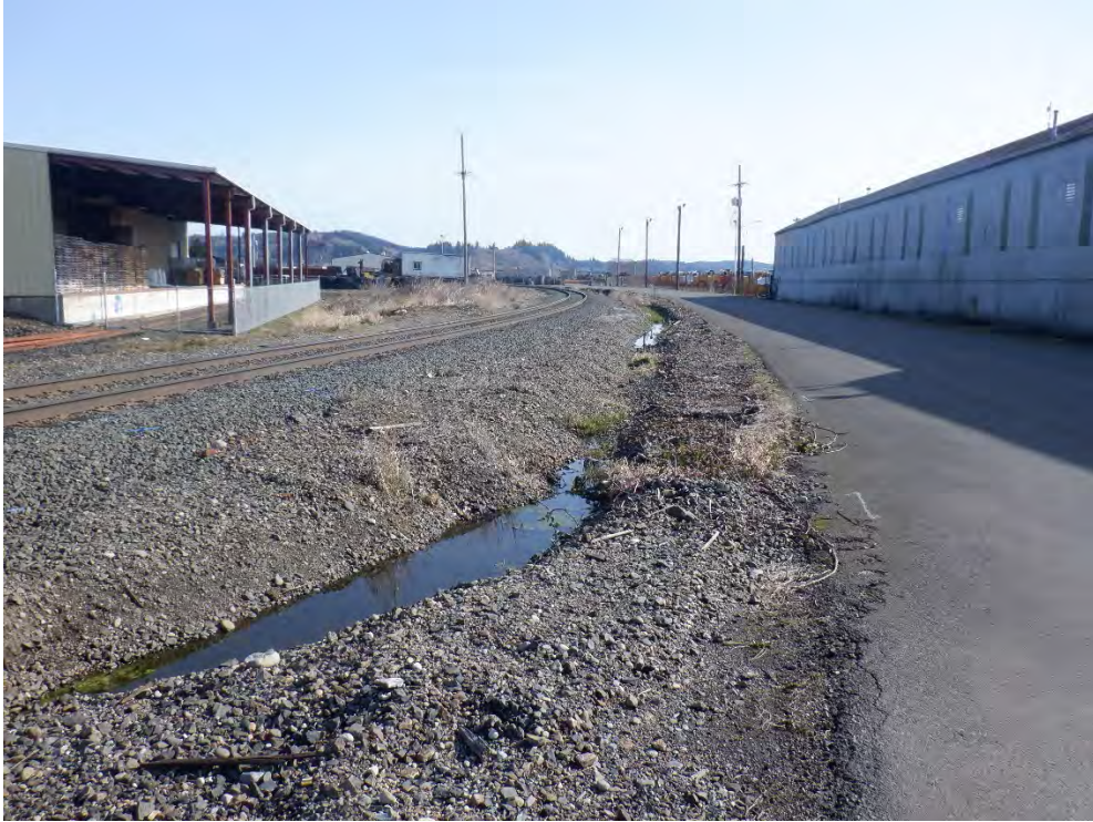
Figure 7 – Formerly identified as Wetland 6 reclassified at Ditch 6. Facing east near intersection of S Monroe St. and W River St.
