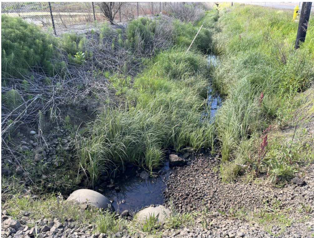
Photo 2: Overview of Wetland 1, south of culverts. Photo taken facing south.
