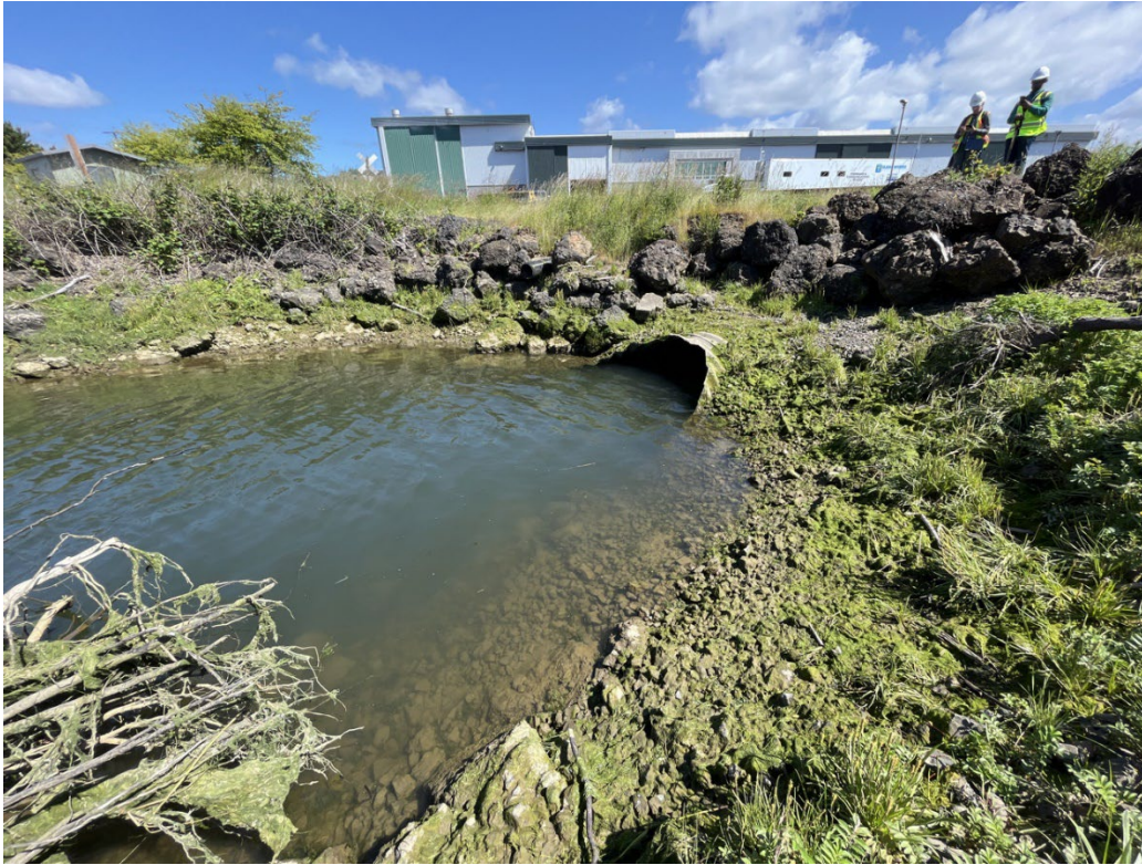
Photo 19: Overview of Fry Creek, south of the culvert. Photo taken facing northwest.
