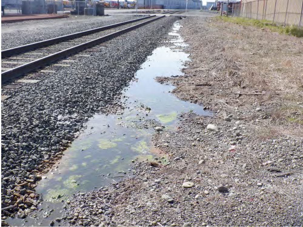
Figure 5 – Formerly identified at Wetland 5 reclassified at Ditch 5. Facing west toward S Washington St.
