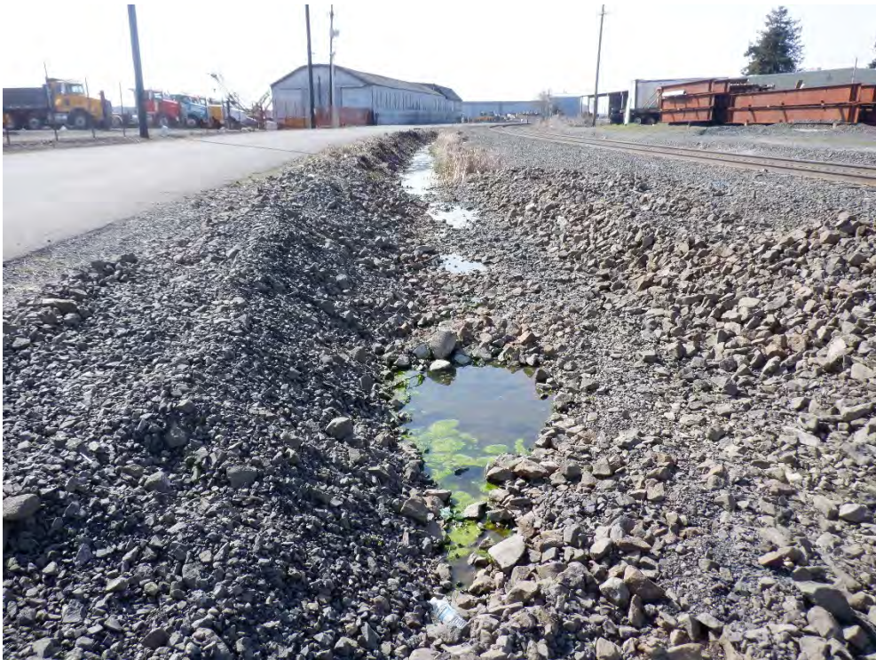
Figure 8 – Formerly identified as Wetland 6 reclassified at Ditch 6. Facing west near intersection of S Washington St. and W River St.
