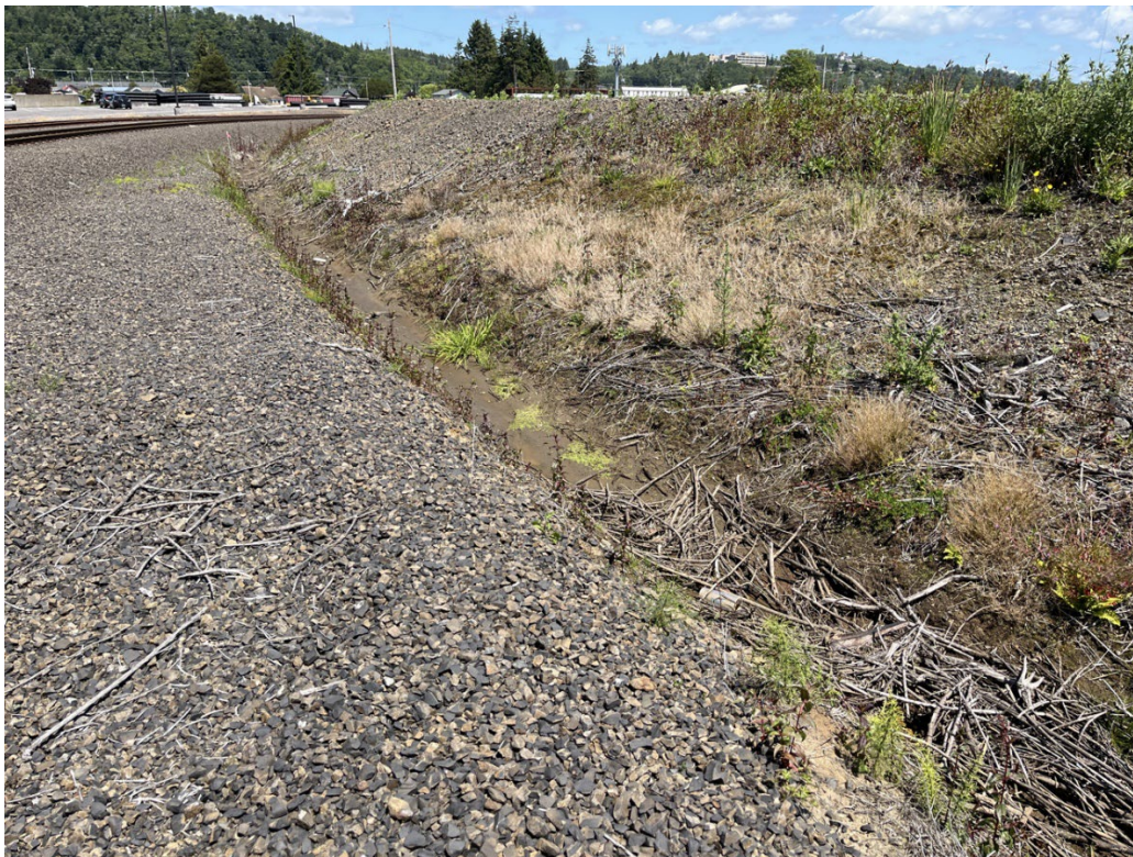
Photo 22: Overview of Ditch 1. Photo taken facing northwest.
