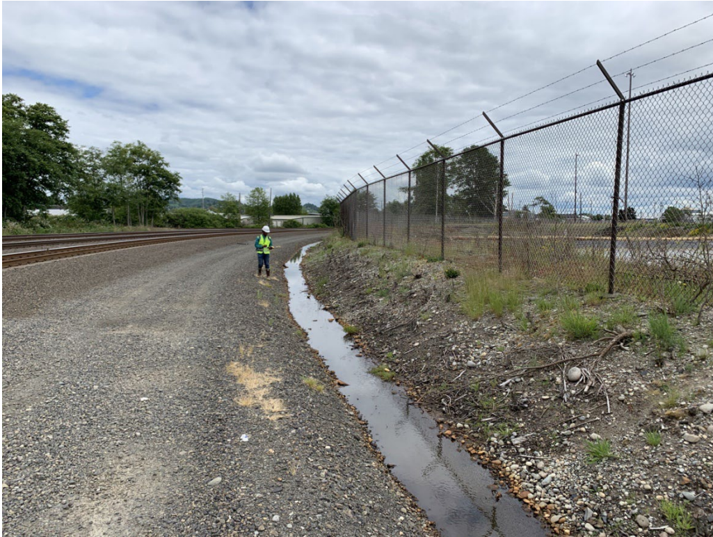
Photo 25: Overview of Ditch 3. Photo taken facing east.
