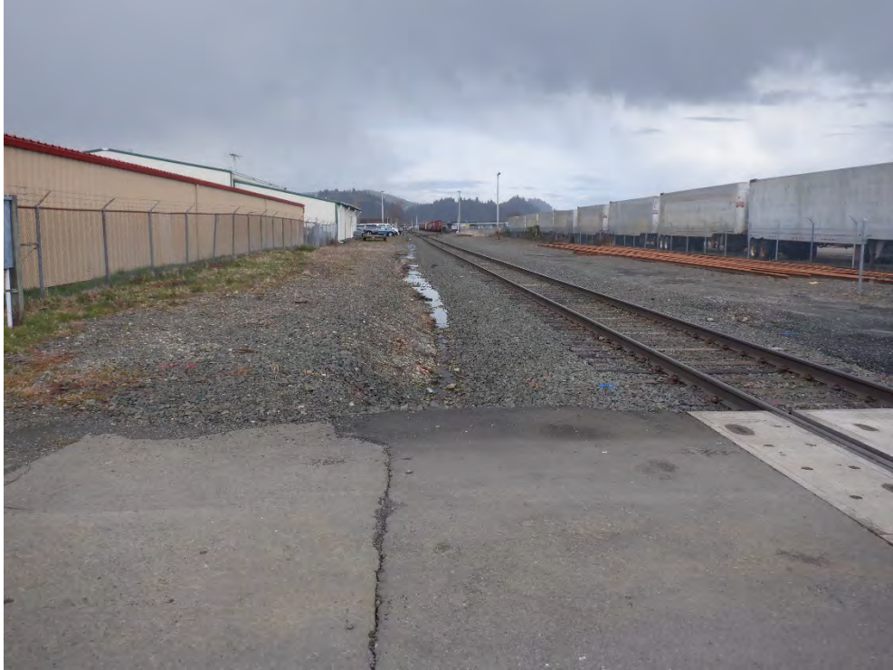
Figure 3 – Formerly identified as Wetland 5 reclassified at Ditch 5. Facing east from intersection of S Washington St and W River St.
